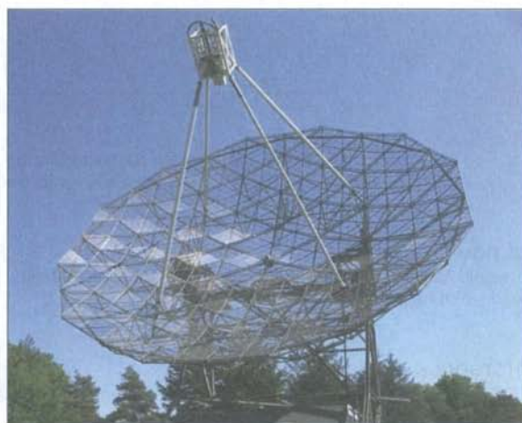
Fig. 11 - D=25 m CAMRAS station antenna
